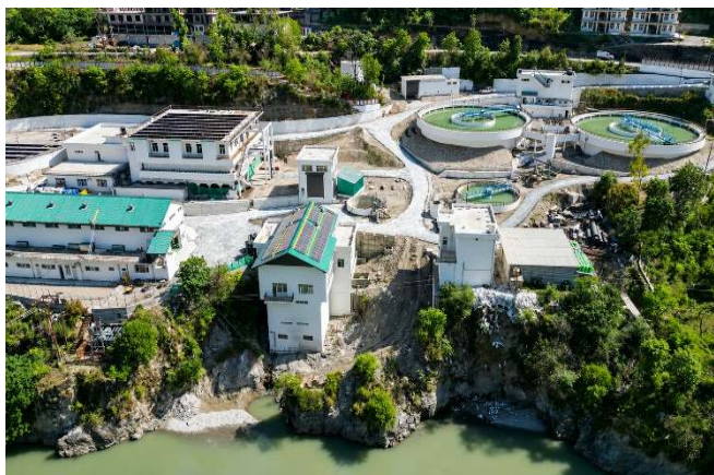
Water Treatment Plant, Shikrodi
